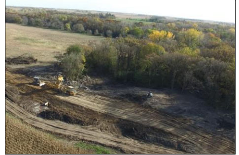
A crew builds a ravine-stabilization berm this fall on Dwane Hull's property in Austin Township near the Cedar River.
