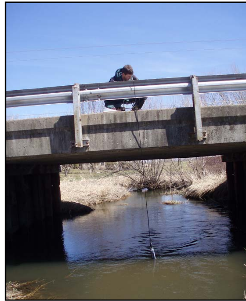
Monitoring on Judicial Ditch #5 at the Mower County 25 Bridge
